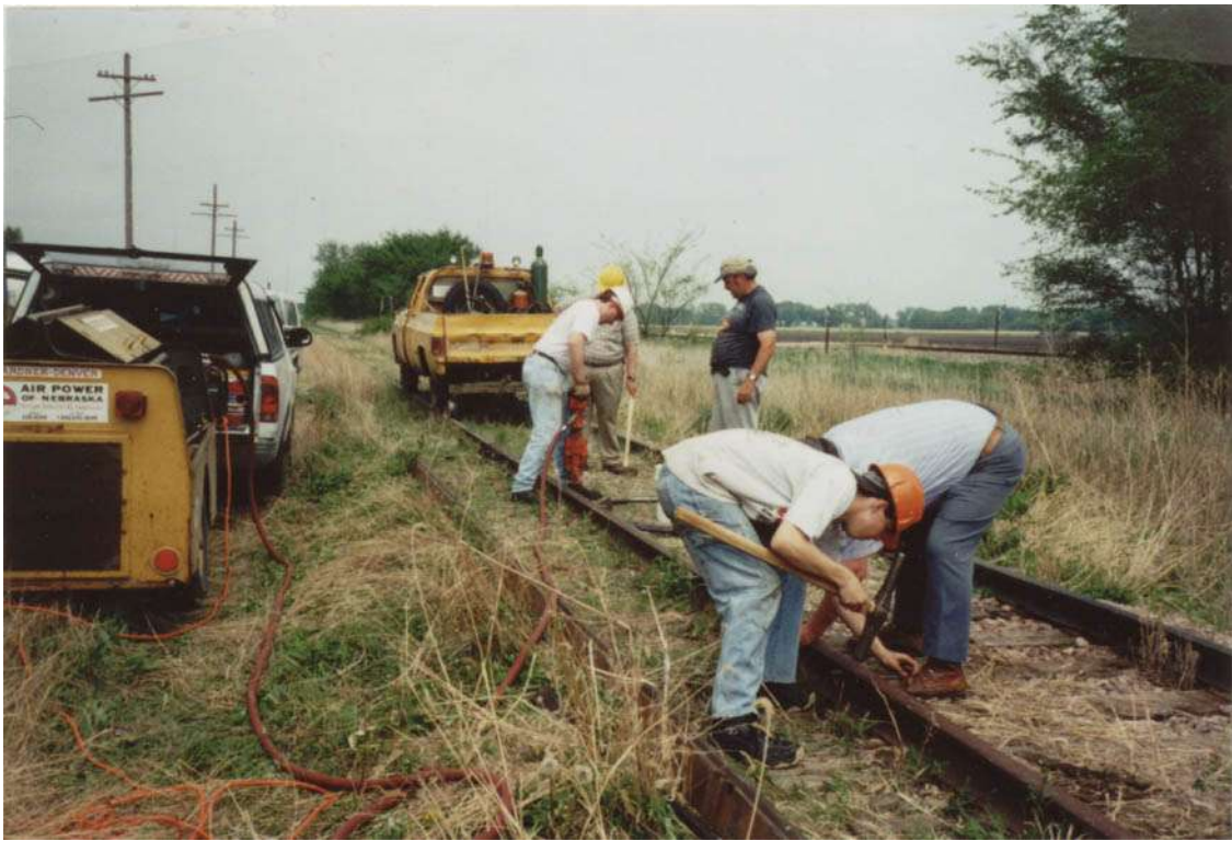
RAILSCENE: Chapter members replacing rail, Nickerson yard, Summer, 1999
