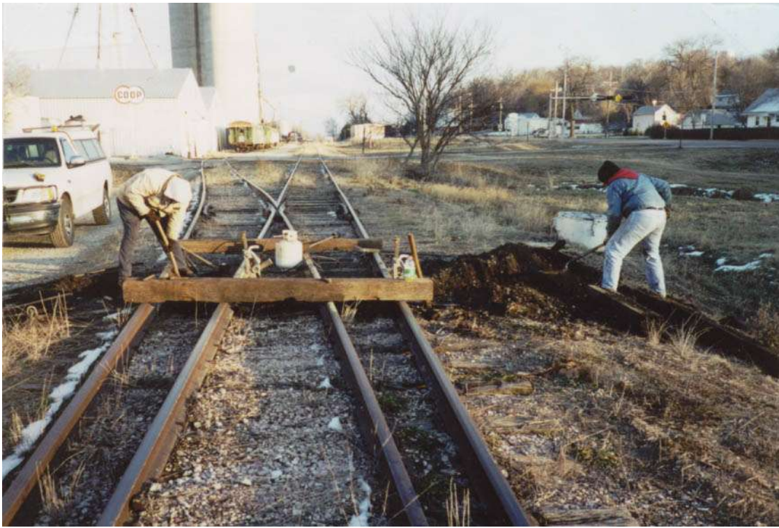
RAILSCENE: Chapter members Allen Schlapfer and George Blessing replacing ties at the west turnout, elevator track, Hooper yard, December, 1999.
