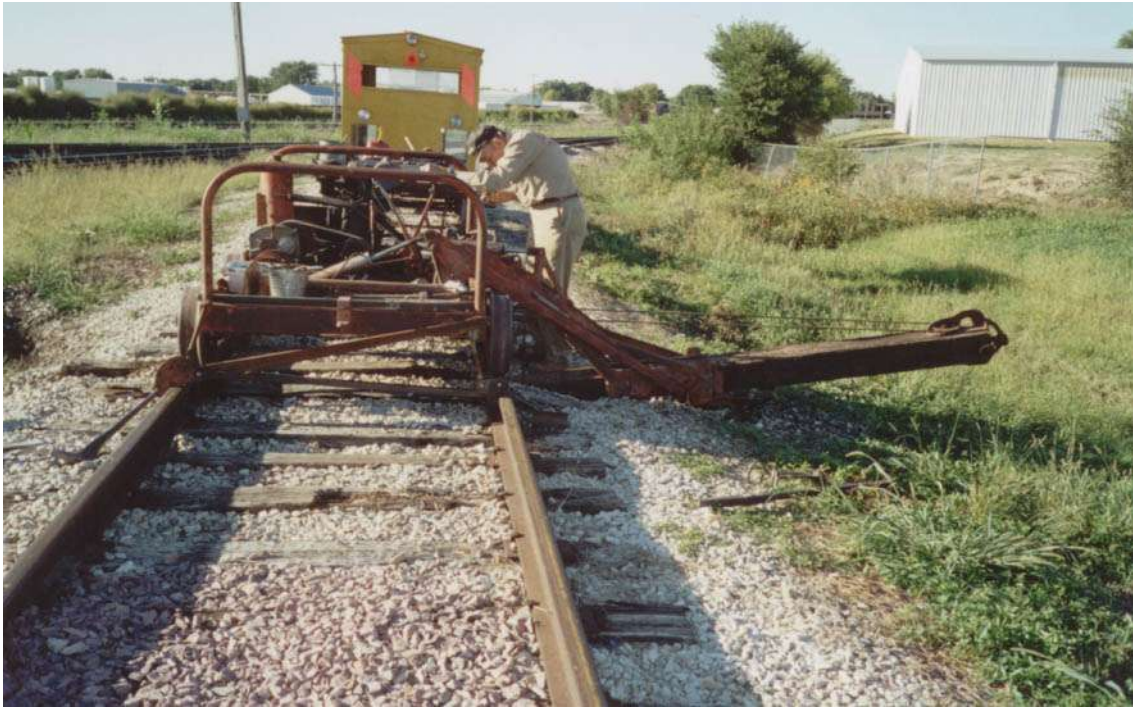
RAILSCENE: Mr. B. H. Hesemann operating the tie replacing unit. As the new tie is pushed under the track (right side of photo), the old tie is forced out (seen emerging from under track left side of photo).
