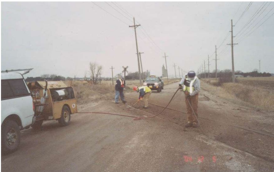
RAILSCENE: Clear Crossing! Al Schlapfer, Erik Mutthersbough, and George Blessing cleaning sand, soil, and debris out of the flangeways at a county road crossing near Fremont on December 5, 2004.
