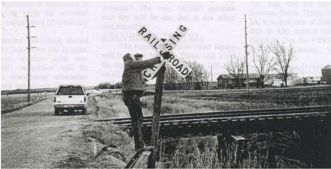
RAILSCENE: "X" marks the spot! This "X" is the spot where the motorist must be alert to look for possible train movements. Volunteer George Blessing installing a replacement county road "crossbuck" on a cold December Sunday!
