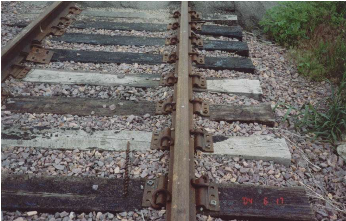
RAILSCENE: Type of construction for the new highway crossings. Screw fasteners attach tie plates and clips hold the rail to the plates providing a durable construction. (story inside - Photo on Iowa Northwestern, Allendorf, IA)
