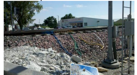
Union Pacific raised track in Missouri Valley, Iowa. The original track level was about at the level of the base of the crossing signal in the photo. Photo by an NRM member.
